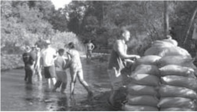
*Volunteers filled, hauled, and placed more 900 sand bags in the creek, creating a temporary dam diversion to allow heavy equipment access to build the retaining wall.*
